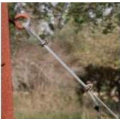
Support wire from post
