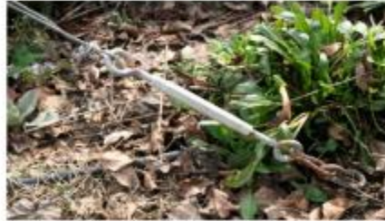
Support wire & turnbuckle attached to earth anchor
