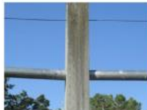
Chain link top rail (hole saw to drill holes)
